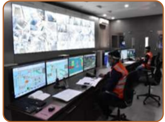
Integrated Control Room
