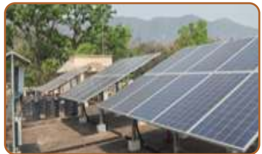
Harnessing solar energy
