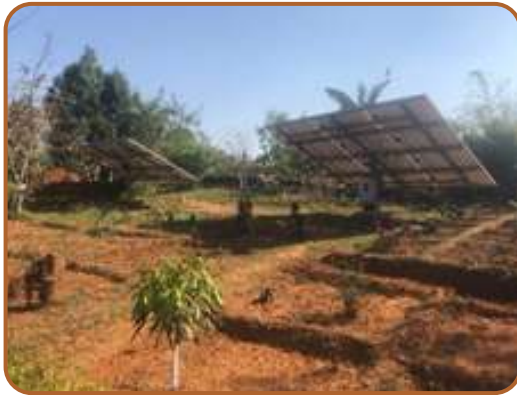
Solar power at nursery
