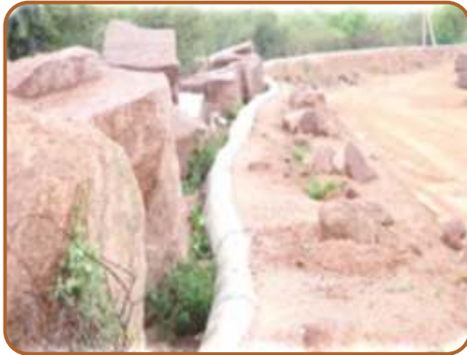
1.5 km pipe line-constructed for water conservation project
