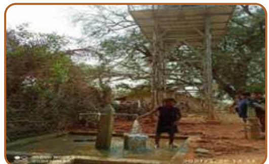
Installation of hand pump for drinking water
