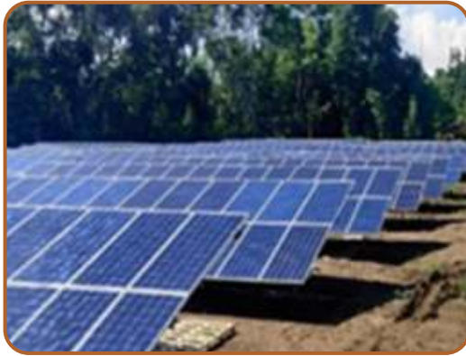
Solar power plant
