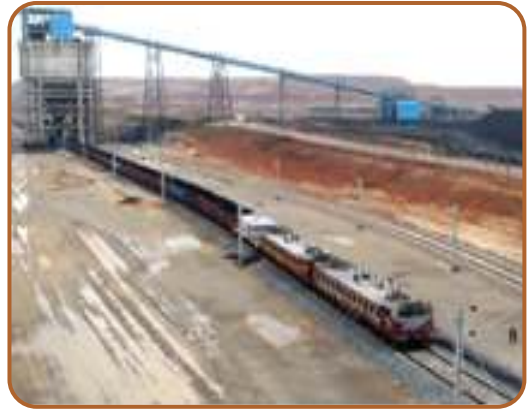
75 km long Private railway line for ore transportation
