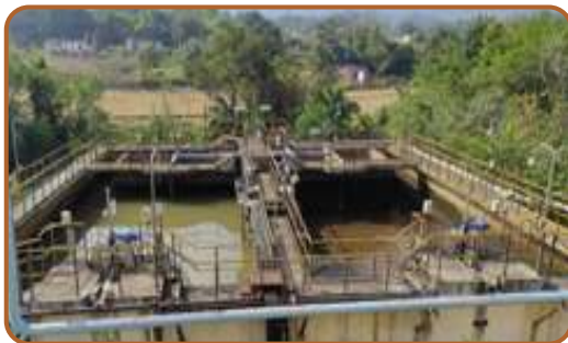
STP of 2 MLD capacity
