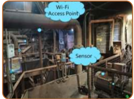
MTR (Maintenance Technology Roadmap) installed on equipment
