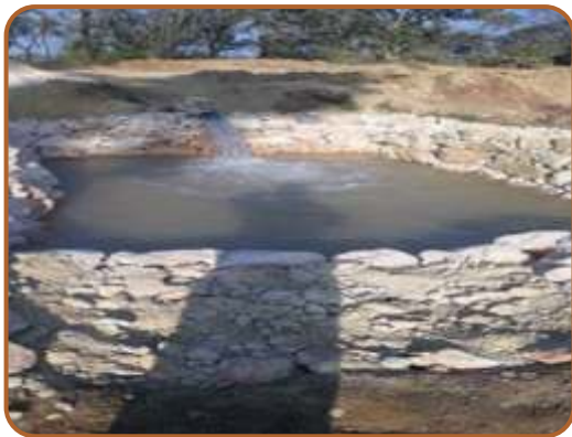
Settling pond for water drainage
