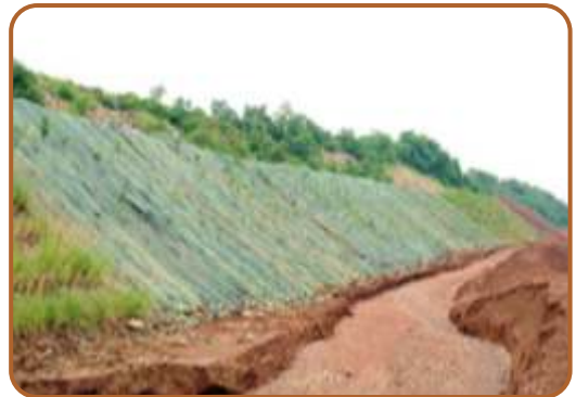
Dump stabilization by coir matting
