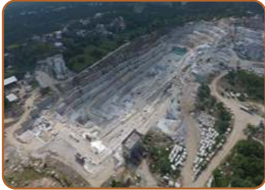
Aerial view of Marble Mine
