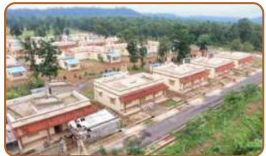
Rehabilitation and Resettlement colony provided by OCPL
