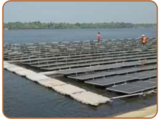
Floating solar plant
