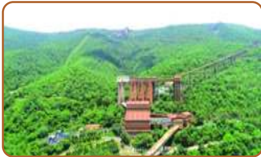
Closed belt conveyor for transporting ore
