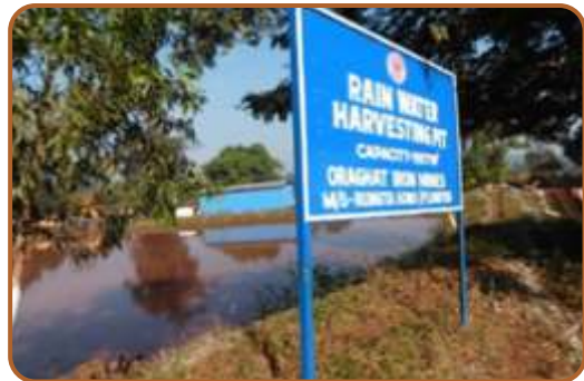
RWH at mines
