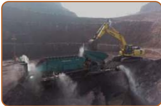
Water sprinkling system at screening plant
