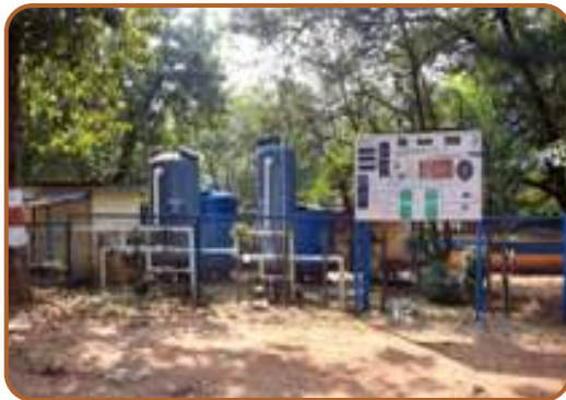
Sewage Treatment Plant
