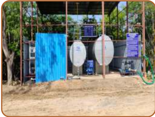
Biodiesel storage and handling
