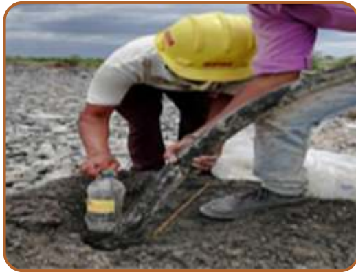
Plastic bottles used for blasting
