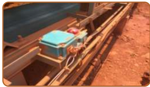
Pull cord switch at conveyor
