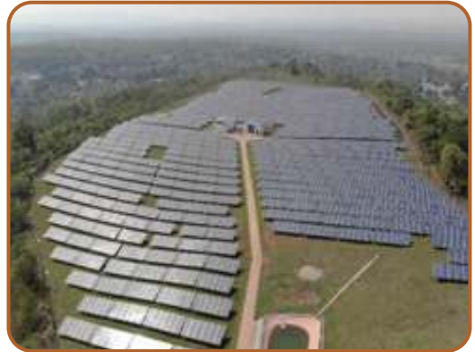
Solar Power Plant of 3MW capacity
