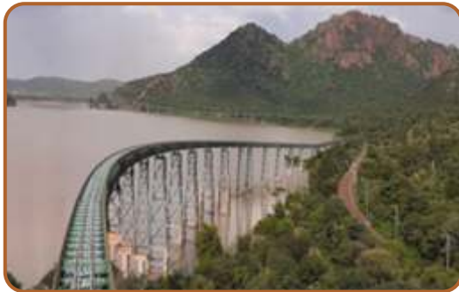
24 km long Pipe Conveyor
